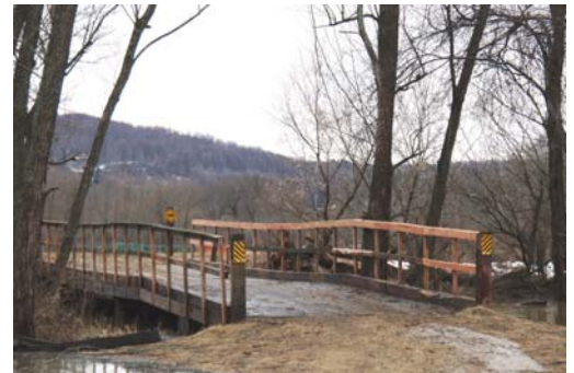
The first bridge installed in Franklinville as part of the Recreational Bridge Project
